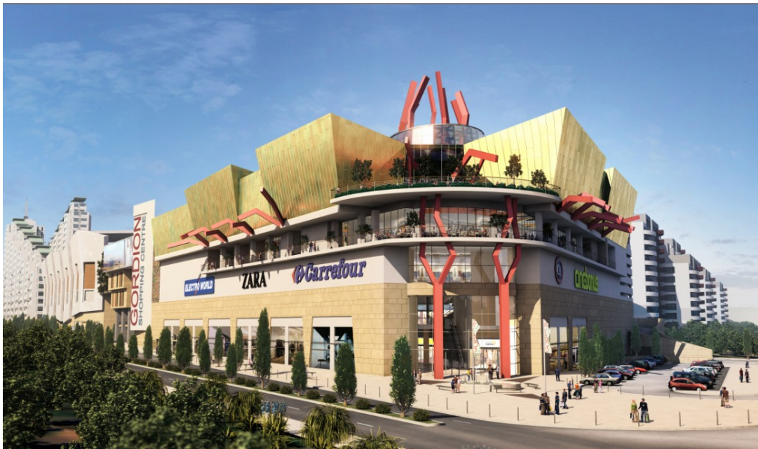
The Gordion Shopping Center will be the first building in Turkey to have a BREEAM certificate.
