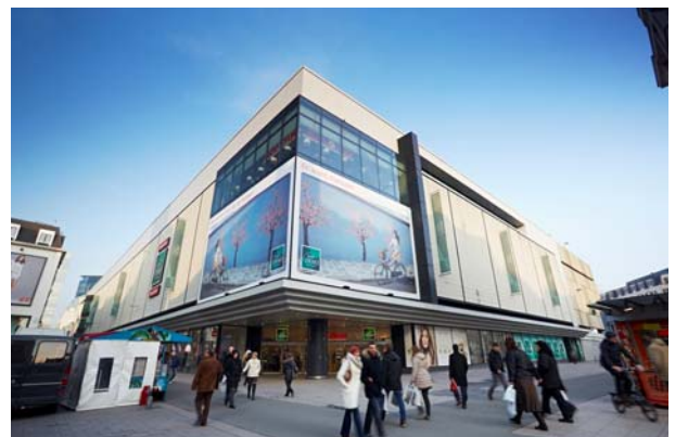
BREEAM In-Use certified: Galeria INNO building in Brussels
