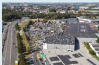
Shopping Cascade, Drogenbos Multi-tenant shopping park
