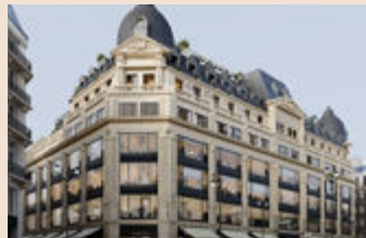
Redevelopment in Progress (ex C&A) - BPM Project 122-126 Rue de Rivoli
