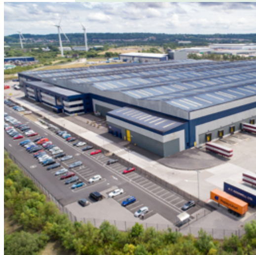
Bristol | The UK Accolade distribution centre
